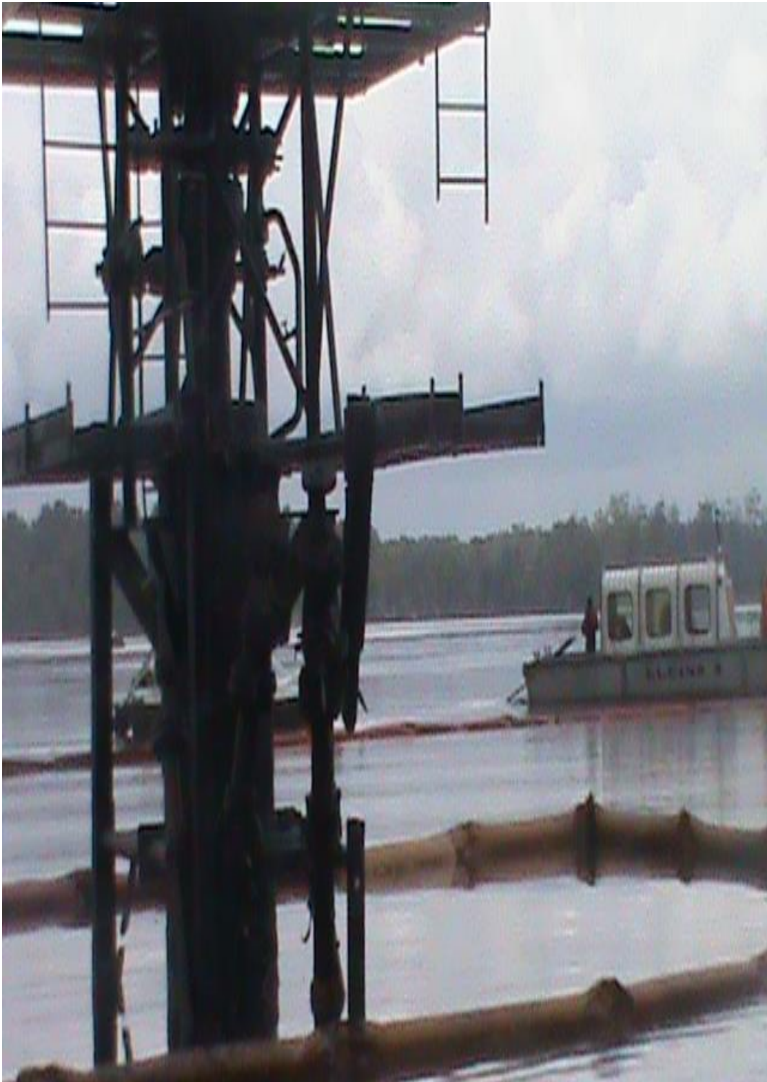
Plate 4.6: NAOC Offshore Oil facility situated inside the sea in Ogulagha Kingdom meant for pumping crude from offshore into Obuguru community
