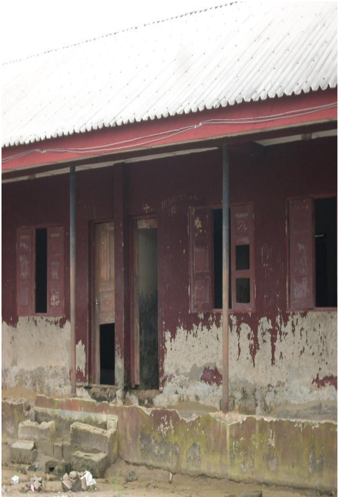
Plate 4.20: NAOC's Donated Primary School in Obuguru community, Ogulagha Kingdom
