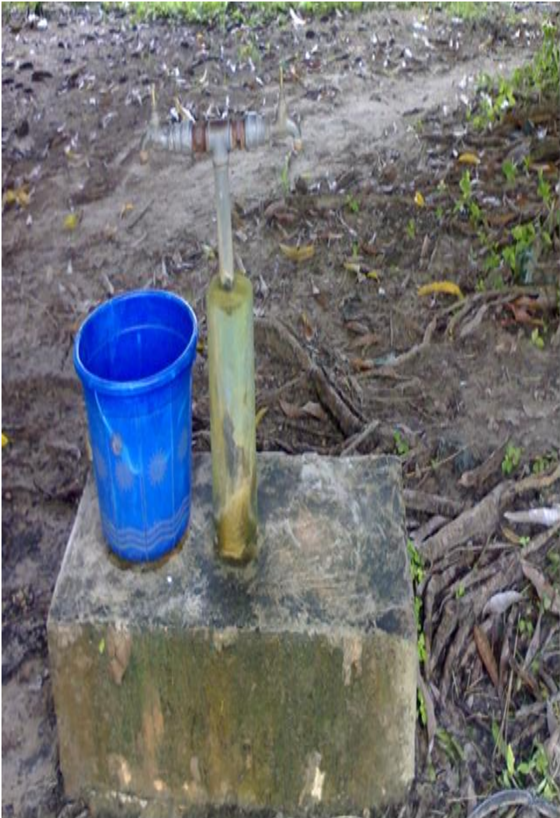
Plate 4.15: This pipe borne water is one of SPDC's developmental intervention in Ogulagha Kingdom.
