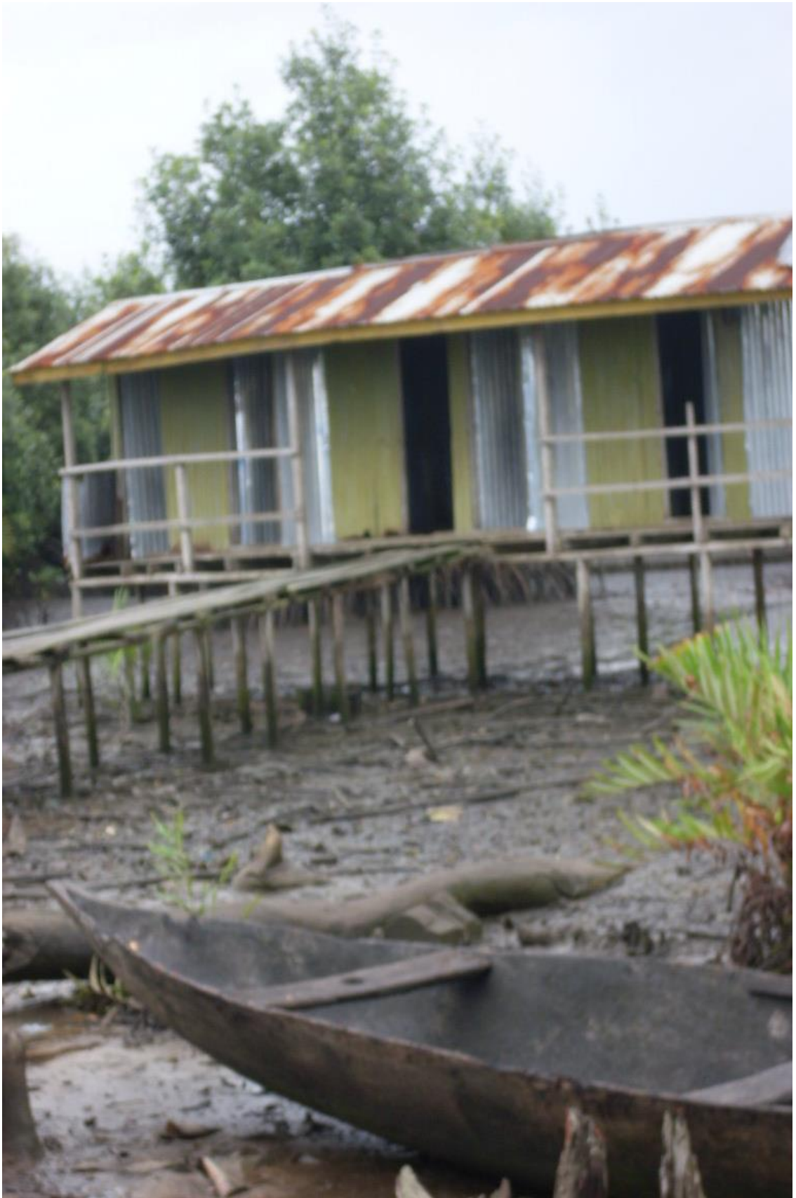
Plate 4.23: NAOC donated public toilet in Obuguru community in Ogulagha Kingdom Source: Fieldwork, 2017
