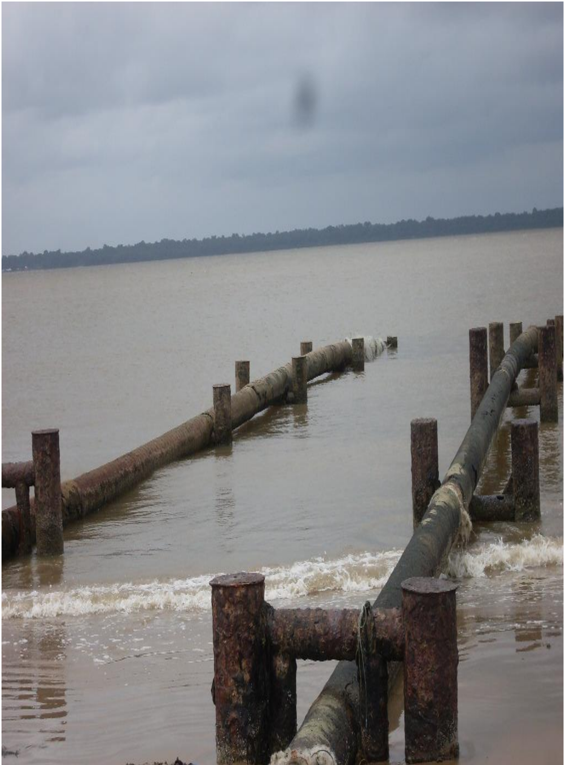
Plate 4.5: Shell's corroded pipes meant for pumping crude from offshore into Yubebe community.
