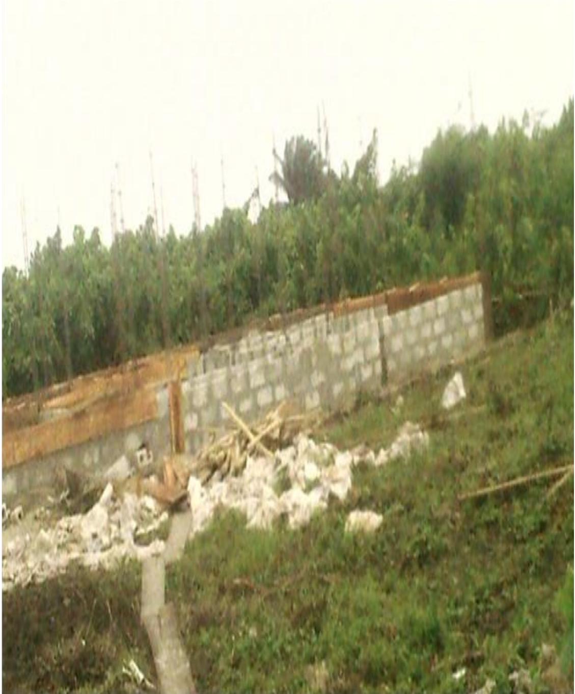
Plate 4.18: SPDC's Primary School Initiative in Youbebe Community (under construction).
