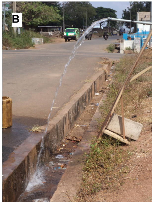
Plates 3.2: Methods of control of water infiltration from groundwater discharge within the vicinities of tested wells. A- Groundwater flow being collected in water containers at Ayete. B- Groundwater flow being drained into concrete drain-line at Igboole in Igboora.
